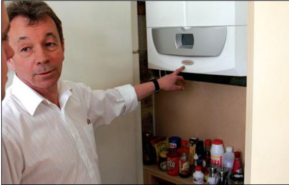
A new Immergas 92 per cent efficient condensing gas combi boiler that meets space heating and hot water needs
