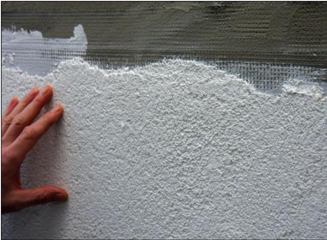
The various layers of the breathable render system that Ecofix installed over the external insulation
