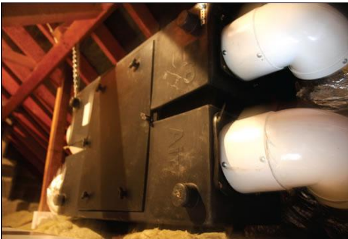
Galway HRV manufacturer ProAir supplied and installed their ProAir 300 system. The unit is listed on SAP Appendix Q and boasts a heat recovery efficiency of 85 per cent
