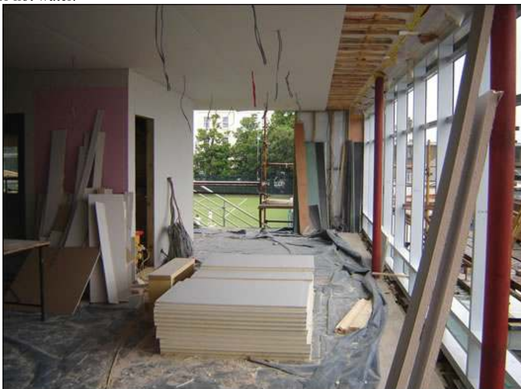
The curtain walling going up, and the ceiling showing insulated plasterboard, battening, and Siga Majpell membrane
