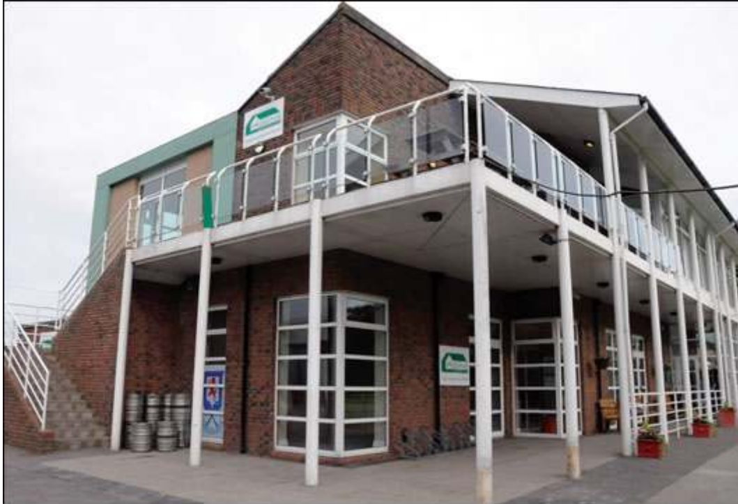
Part of the original balcony has been retained, and part has been enclosed inside the new glazed curtain walling
