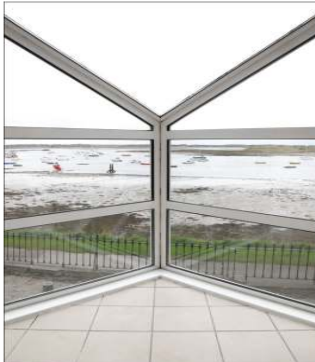
The glazed curtain walling with a centre-pane U value of 1.2 W/m 2 K provides excellent views over the harbour to the north, and over the tennis courts to the south
