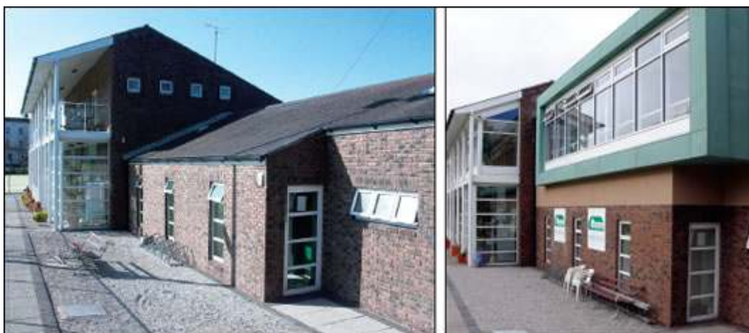
Before and after shots of the front facade, showing the new glazed extension with green copper cladding over the changing rooms
