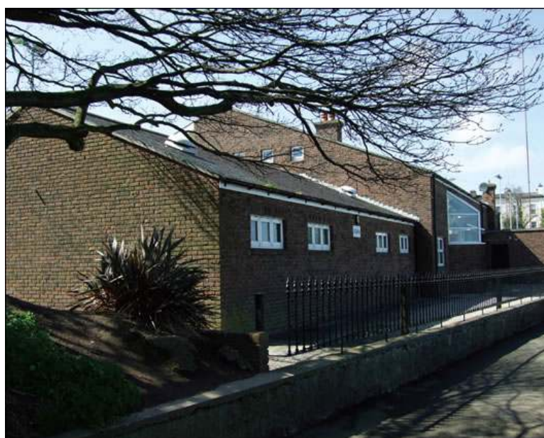
A rear view showing both sections of the building before the upgrade
