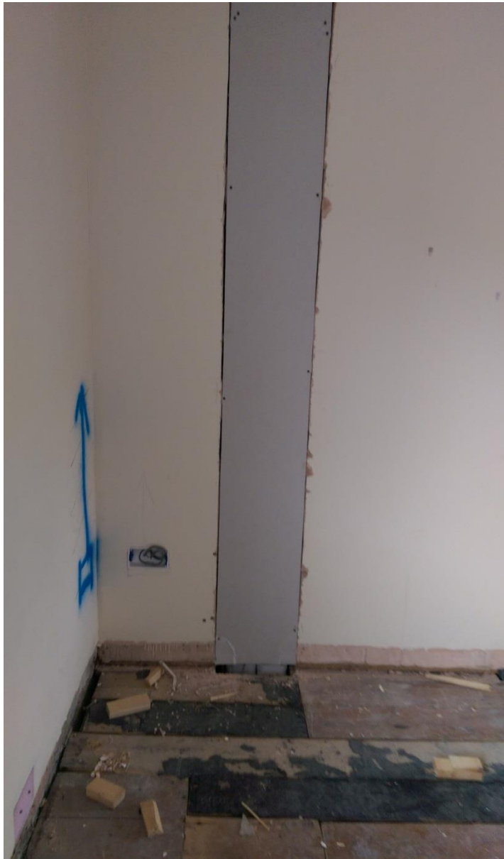
4 Wall with duct in stud ready to be plastered
