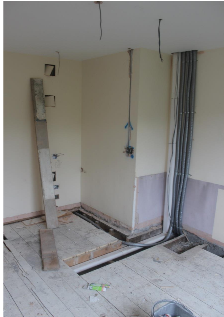
1 Ducts serving ground floor room in the back of a wardrobe
