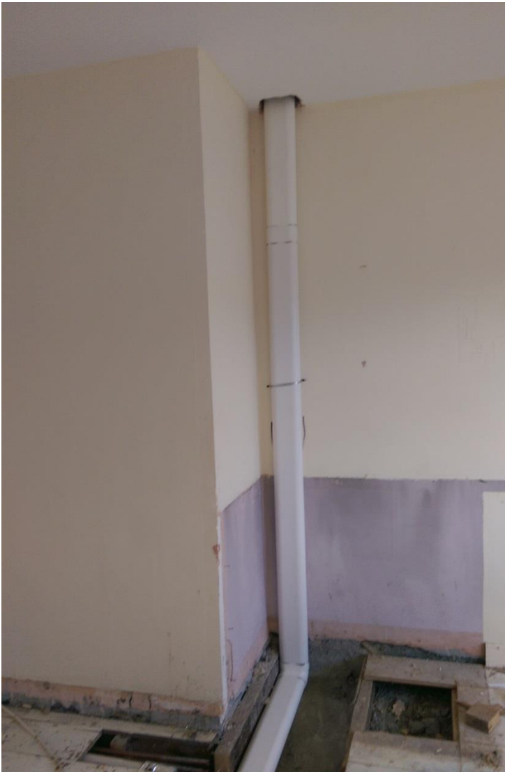
1 Ducts serving ground floor room in the back of a wardrobe
