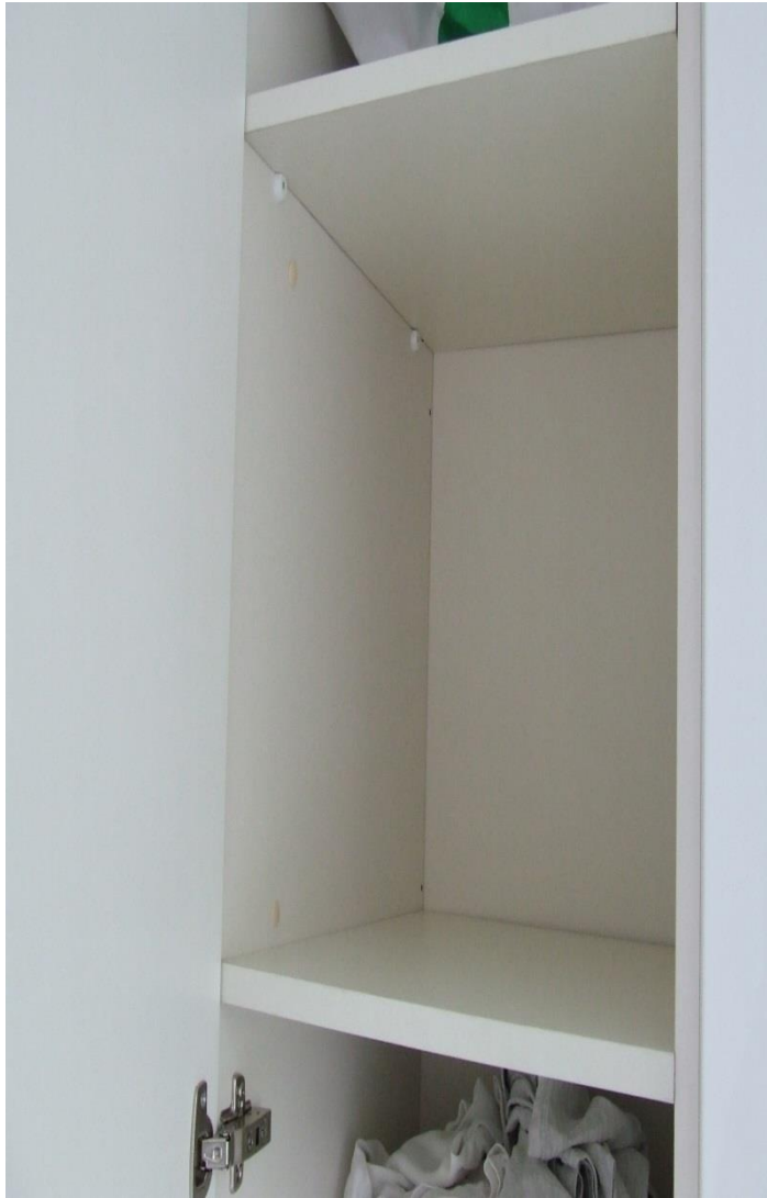
7 Ducts hidden in wardrobe and boxed ducts
