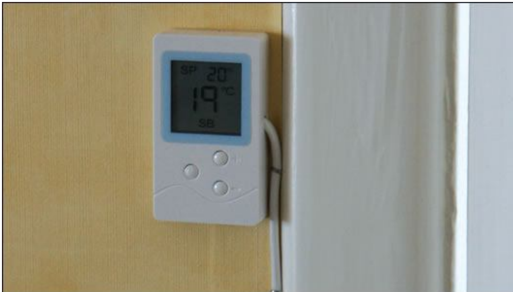
The Radmaster system features simple controls in each room that enable the householder to turn the temperature up or down
